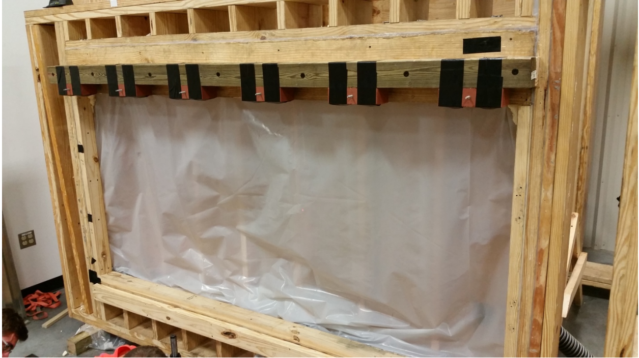
Figure 8. Configuration B1 (without structural panel installed). Photo taken during construction. The bottom boundary condition (not shown) mirrored the top (shown)
